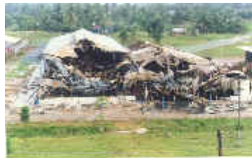
This rattan furniture factory was destroyed by a contractor working unsupervised on a weekend. He was welding on one side of a wall and ignited foam on the other side. The equipment left behind can be seen on the right.
